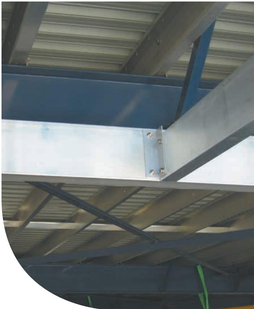
Engineered PERMALITE® aluminium purlins and bridging provide a lightweight, high strength option to extend the corrosion resistant qualities of marine grade aluminium beyond the external cladding and windows to include support framing as well.
