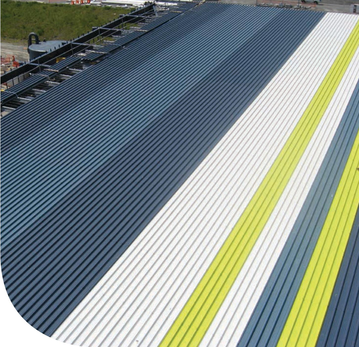
PERMALITE® products are made from marine grade aluminium, roll-formed to produce high performance cladding or purlins with an exceptional combination of strength and light weight.
