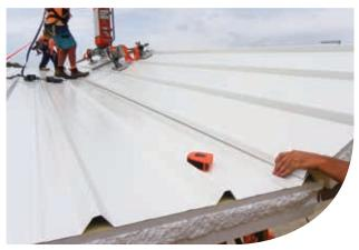
Figure 5.4 ALSULATE-125® panels after joining
