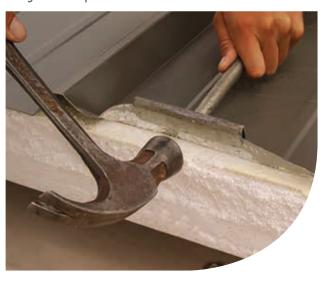
Figure 4.4: Turn down all the roof pans at the gutter end using the turn down tool
